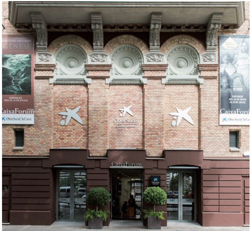
CaixaForum Lleida commemorated the 100th anniversary of its building, filled with Art Nouveau details.
